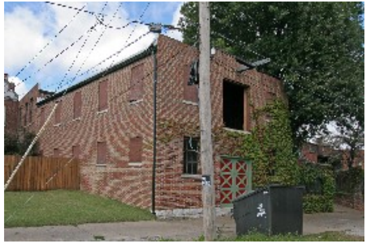
The rear stable building viewed from the alley.
